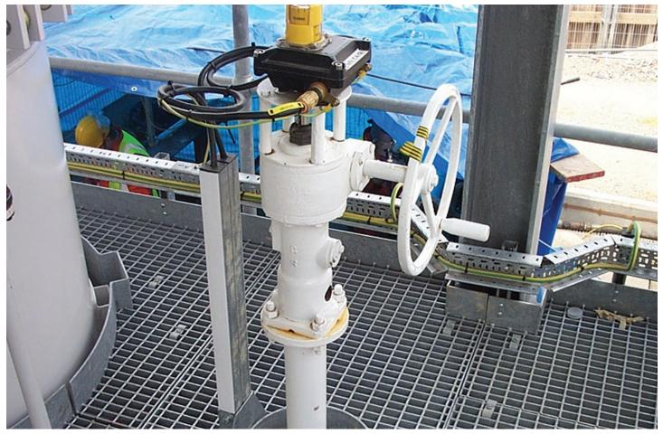
GENERAL VALVE Twin Seal plug valve fitted with enclosed limit switches.
